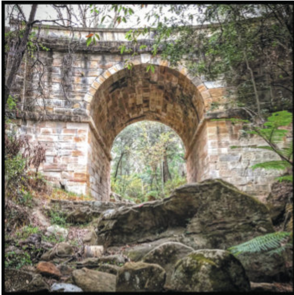
Glenbrook, New South Wales, Australia
